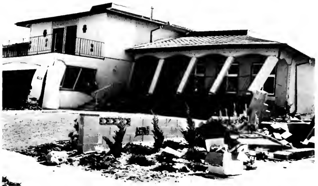
Photo 14. Two-story, split-level, residential structure (Almeiz Street) which sustained damage due to insufficient lateral support provided by ground garage opening and collapse of cripple supports under single-story portion. Courtesy of the City of Los Angeles Department of Building and Safety.
